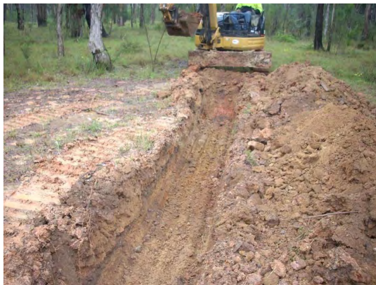
Photo 48. Photo showing location of trench, T2B
